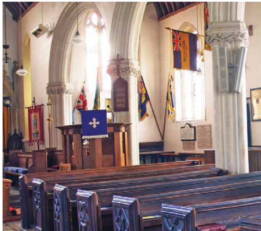
Fig. 6. Two of the arches of the arcade. Both the piers were taken down and rebuilt in 1845.
