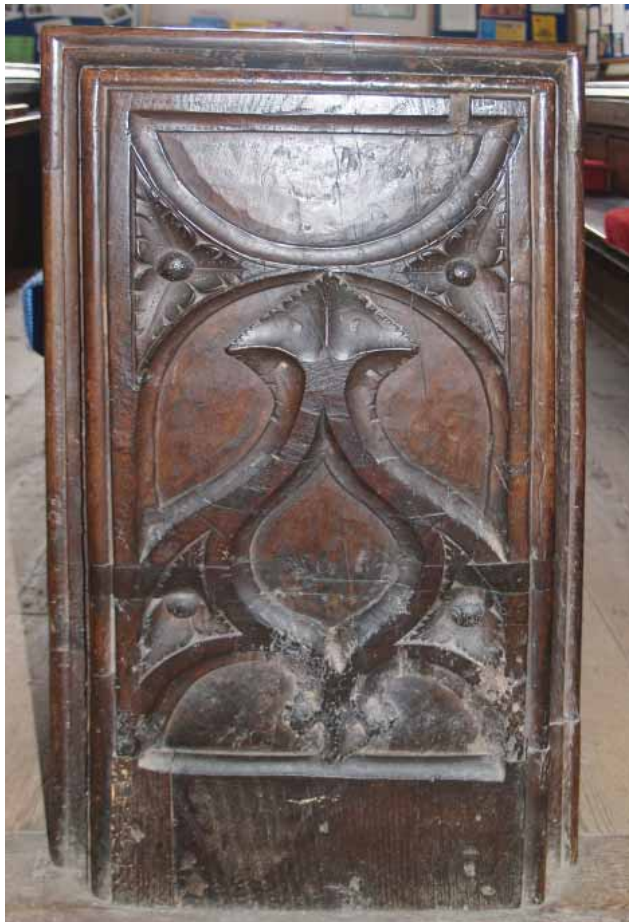
Fig. 15. The scarring on this bench end shows that it once had a flap or sliding seat attached, projecting into one of the aisles when in use.
